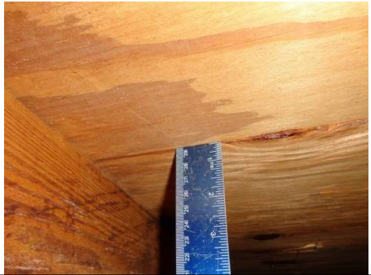
Roof Deck Thickness
