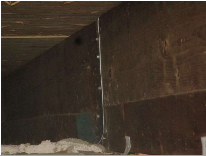
Roof To Wall Connection
