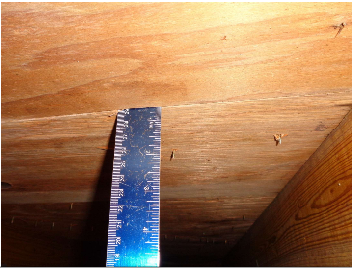
Roof Deck Thickness
