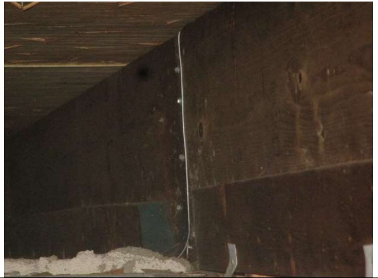
Roof To Wall Connection
