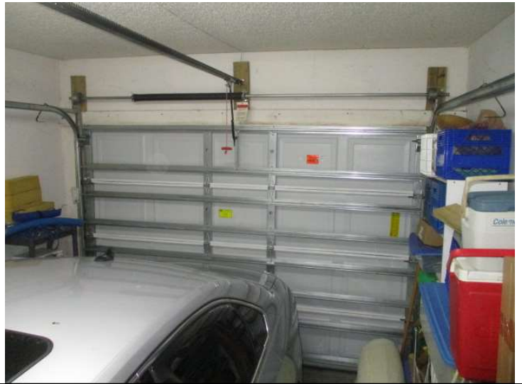
Exterior Opening Protection
