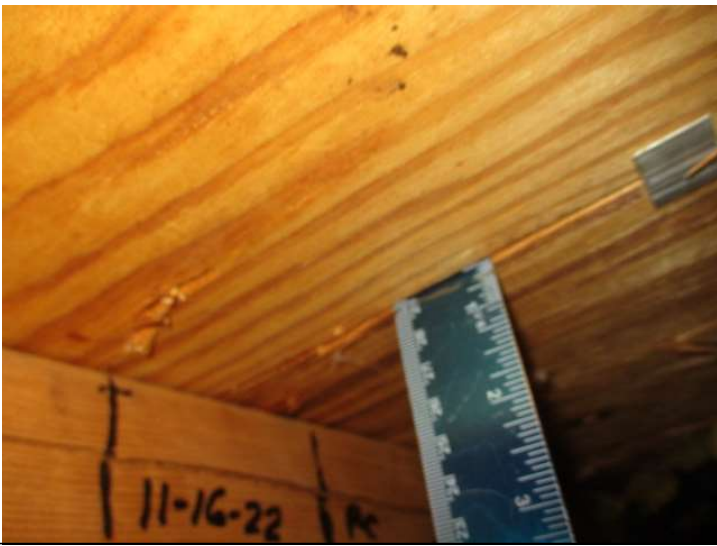
Roof Deck Thickness
