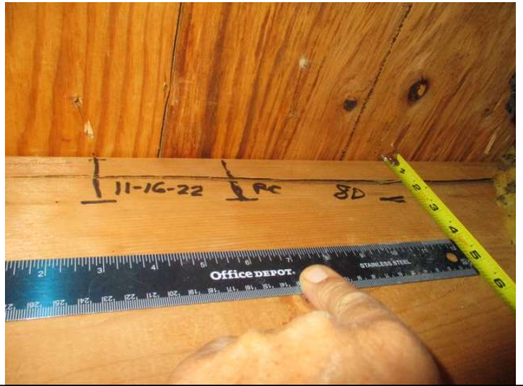
Roof Deck Fastener Spacing
