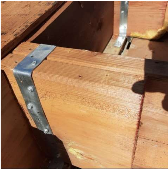
Roof To Wall Connection
