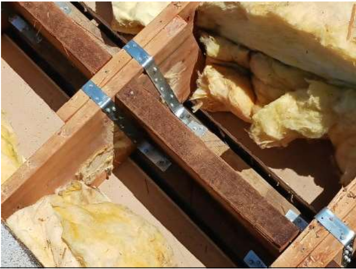
Roof To Wall Connection
