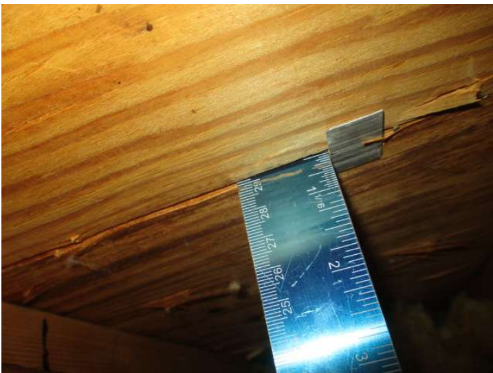
Roof Deck Thickness
