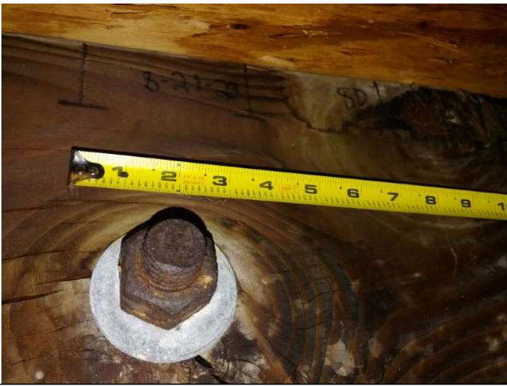
Roof Deck Fastener Spacing
